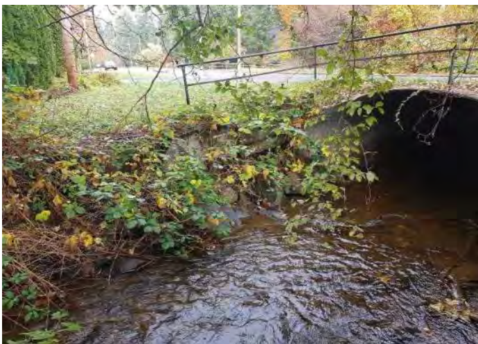
Photo 2, Upstream of culvert, undermining and rotation of gabion basket visible on right bank.
