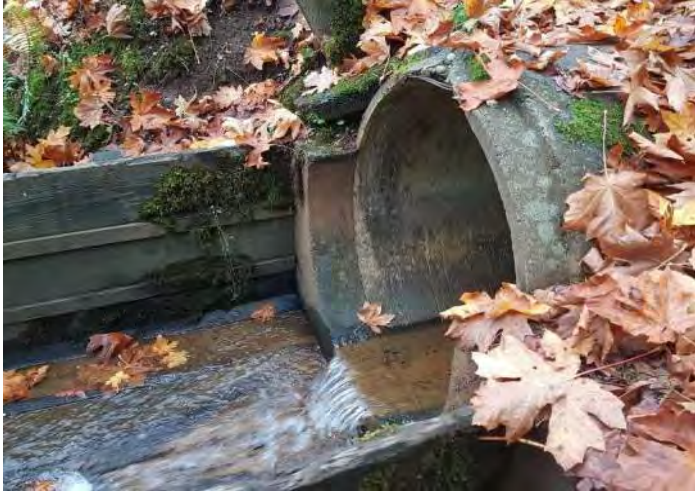
Photo 1, Concrete stormwater pipe flowing into timber flume.
