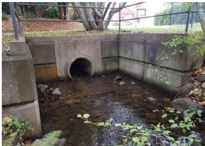
Photo 3, Culvert outlet.
