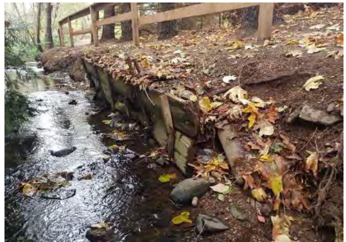
Photo 2, failing wall looking upstream.
