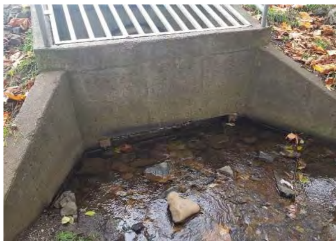
Photo 2, Culvert inlet.
