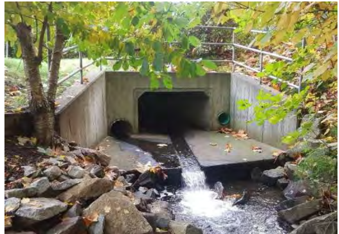
Photo 4, Outlet of Culvert and other pipes, riprap bank protection is visible.
