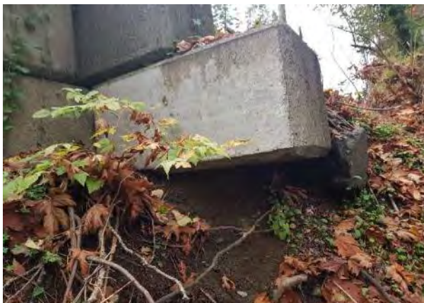
Photo 5. Undermined lock block on left bank at outlet structure.
