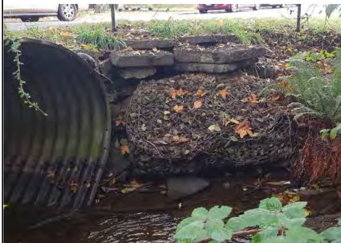
Photo 3, Upstream of culvert, close up of overturning gabion on the right bank.
