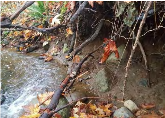
Photo 3, Erosion of right bank downstream of culvert.
