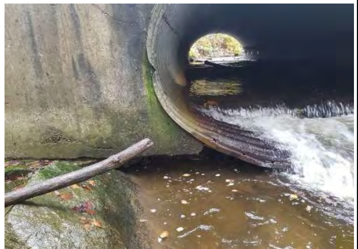
Photo 4, Erosion undermining culvert headwall structure to right of outlet.
