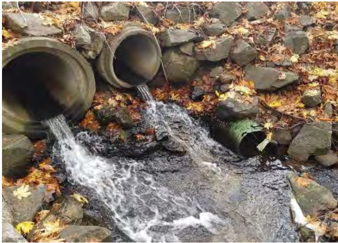
Photo 1, Culvert outlets and storm outlet, mild erosion visible.
