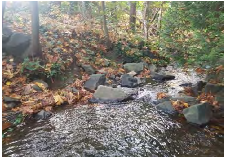
Photo 4, Downstream of culvert outlets, mild erosion on left hand bank visible.
