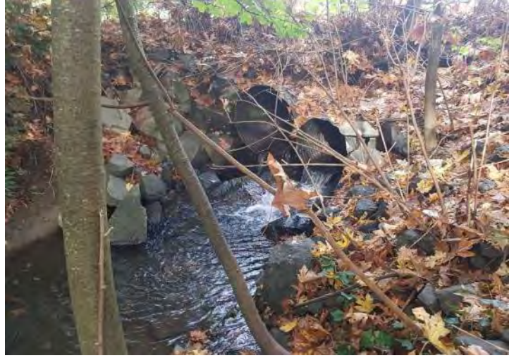
Photo 2, Culvert outlets, erosion visible.
