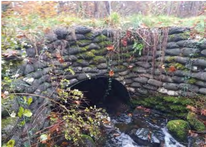
Photo 1, Culvert Inlet, concrete bag wall.
