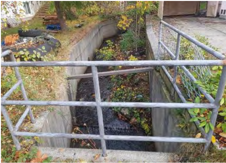
Photo 1, up stream of culvert, concrete walls and bracing visible.
