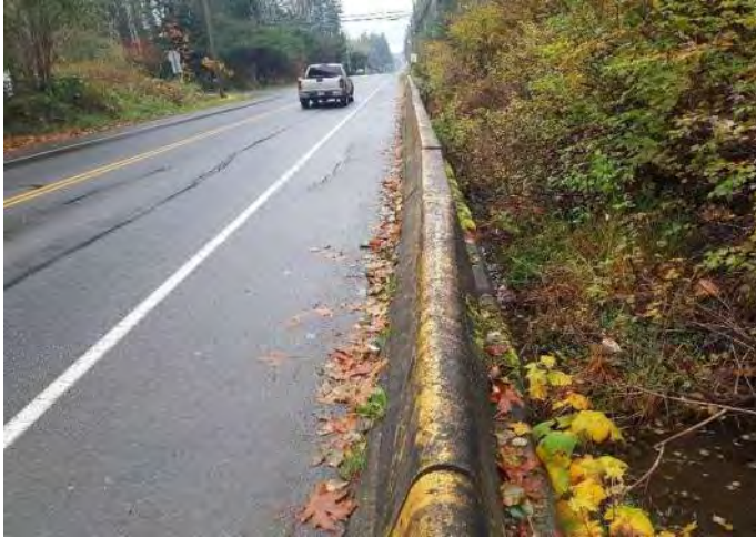
Photo 1, Roadway with creek, cracking on pavement visible.
