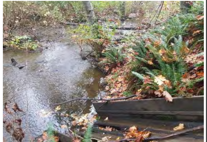
Photo 2, Failure point of timber flume with water leaking onto bank, erosion is visible on the bank.
