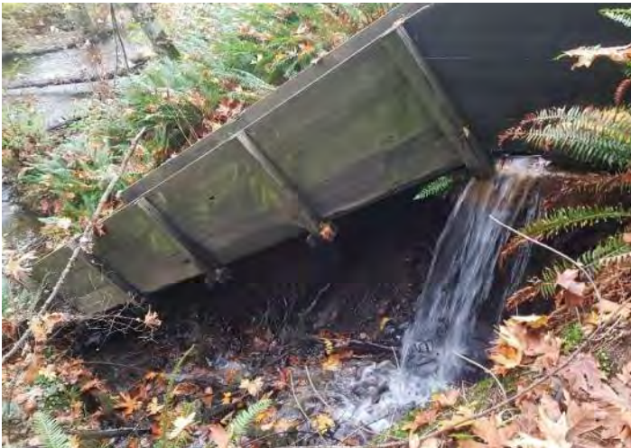
Photo 3, Failure point of timber flume with water leaking onto bank, erosion is visible on the bank.
