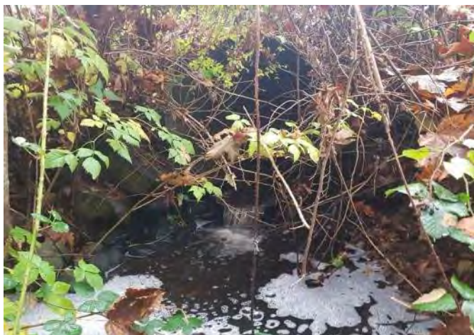
Photo 3, Culvert outlet, drop in channel visible.
