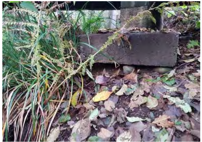
Photo 4, undermining on left bank abutment.
