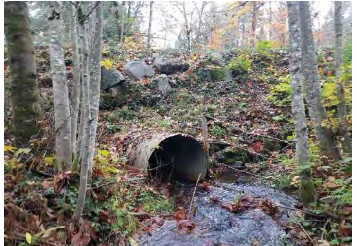
Photo 2, Culvert inlet, dry stack boulder armouring visible on embankment slope.
