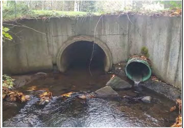
Photo 4, outlets of culvert and storm drainage.
