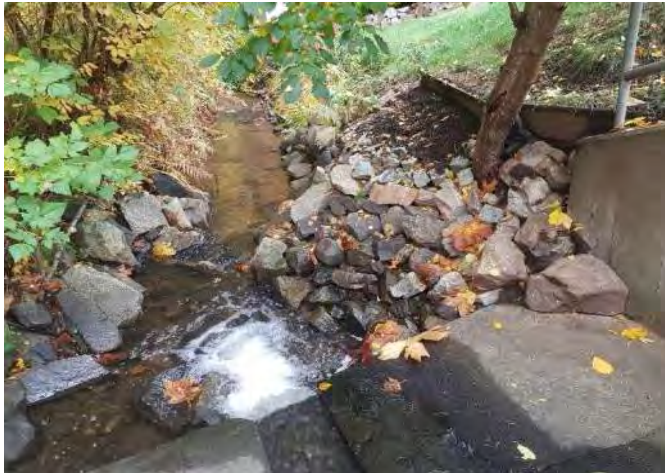
Photo 3, Downstream of Culvert outlet, riprap and channel base visible.
