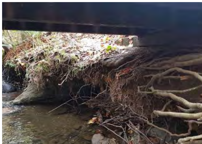
Photo 2, Left bank undermining, bridge abutment visible.
