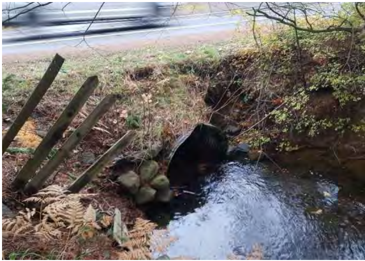
Photo 5 , Downstream culvert outlet, erosion visible on left bank.
