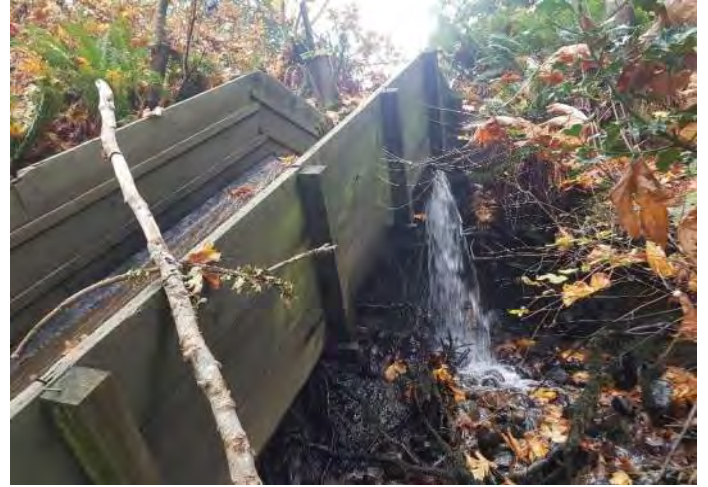
Photo 2, Failure point of timber flume with water leaking onto bank, erosion is visible on the bank.
