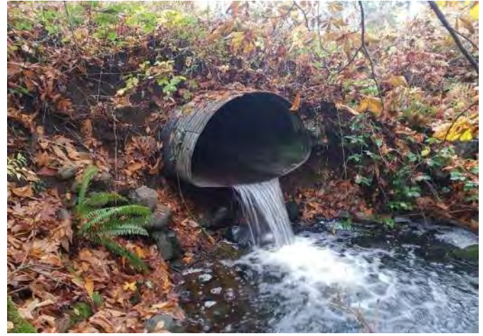
Photo 2, Culvert outlet, erosion of embankment and undermining of culvert visible.
