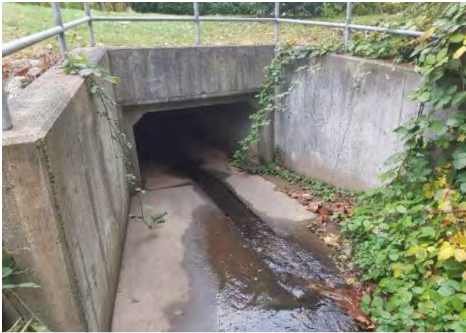
Photo 1, Inlet of Culvert.
