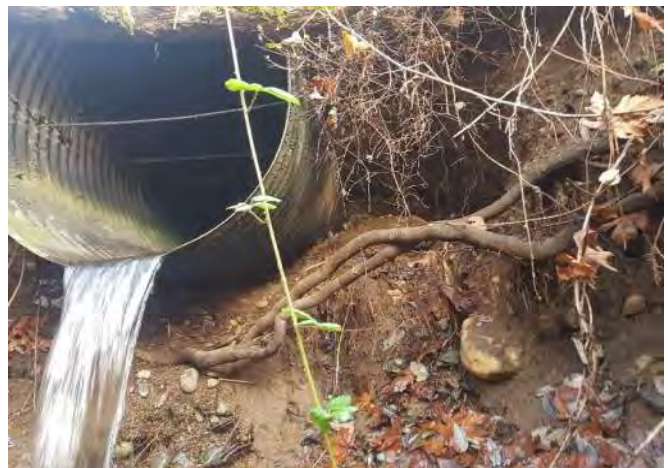
Photo 2, Erosion around culvert outlet, undermining culvert and embankment.
