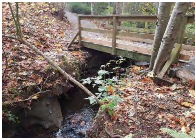
Photo 1, Pedestrian bridge and left bank undermining visible.
