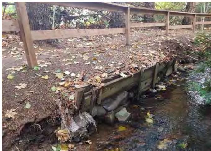
Photo 3, failing wall looking downstream.
