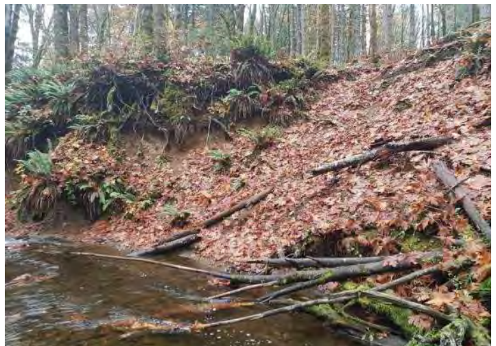
Photo 4, Right bank erosion. Collapsed crest at right side of photo.
