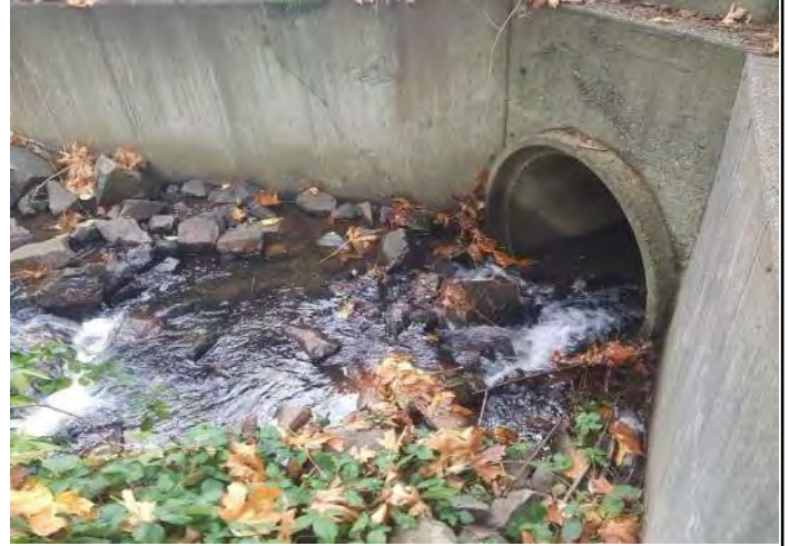
Photo 2, Inlet of culvert.
