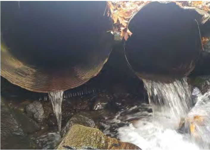
Photo 3, Erosion undermining culvert outlets.
