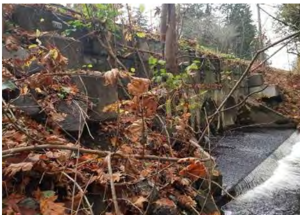
Photo 3, Downstream of culvert, undermining of left and right bank lock block walls visible.
