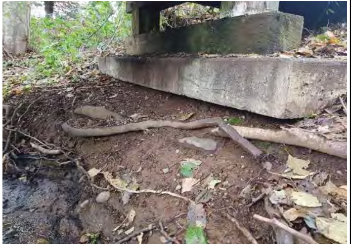
Photo 2, Right bank abutment undermining.
