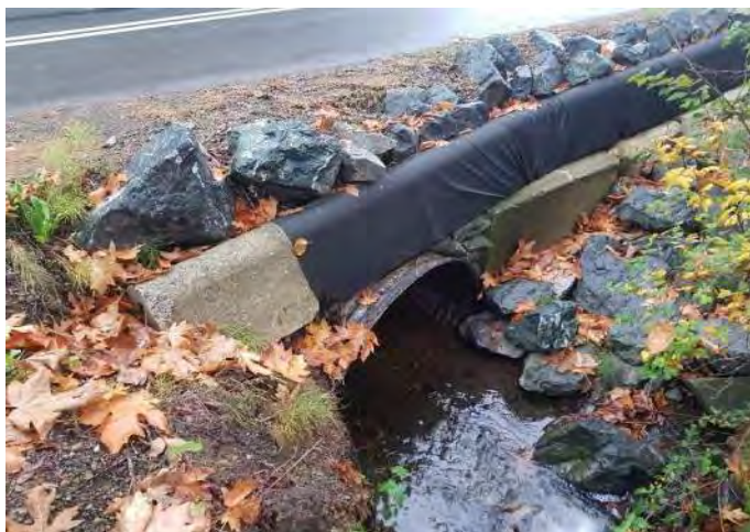
Photo 2, Culvert inlet and headwall.
