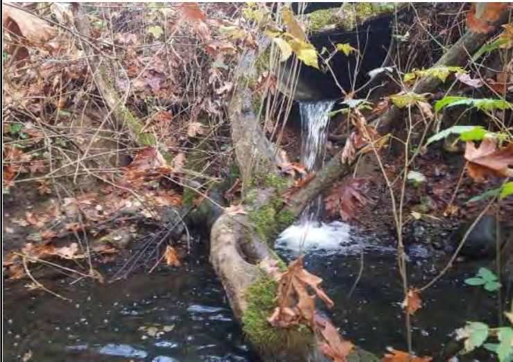
Photo 5, Culvert outlet with 1.5m drop into pool, erosion is visible underneath culvert.
