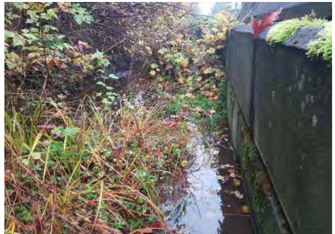
Photo 2, Lock block wall making up left bank of creek.
