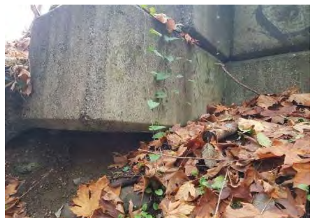
Photo 6. Undermined lock block on right bank at outlet structure.
