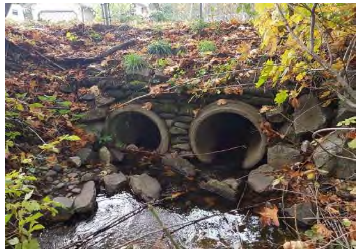
Photo 4, Culvert inlets, concrete bag wall and riprap visible.
