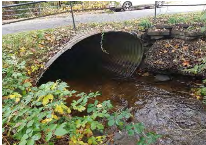
Photo 2, Upstream of culvert, undermining and rotation of gabion basket visible on right bank.
