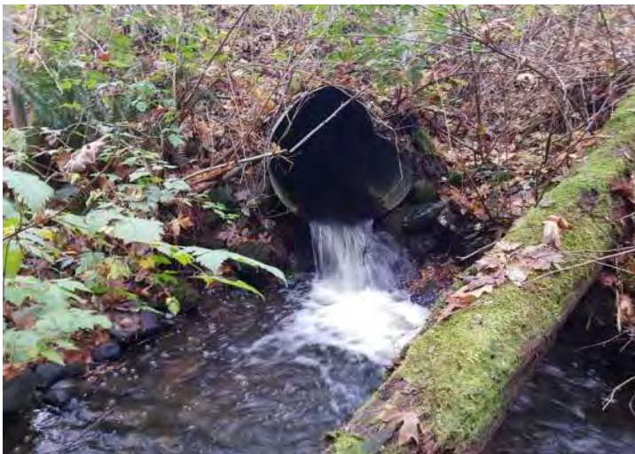
Photo 3, Culvert outlet, mild erosion visible.
