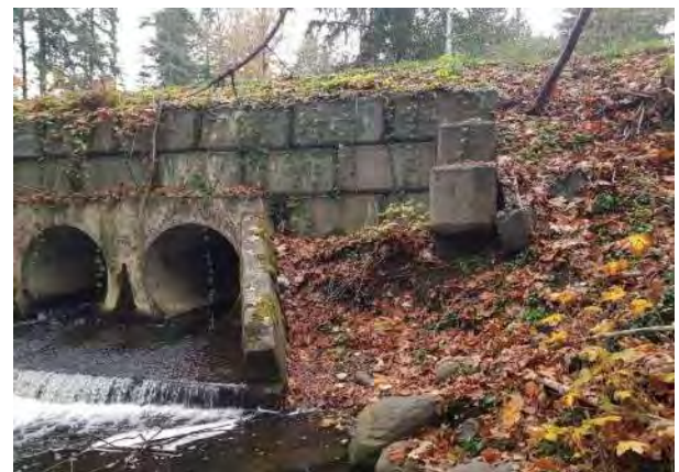
Photo 4, Severe undermining of left bank lock block wall visible. Outlet structure.
