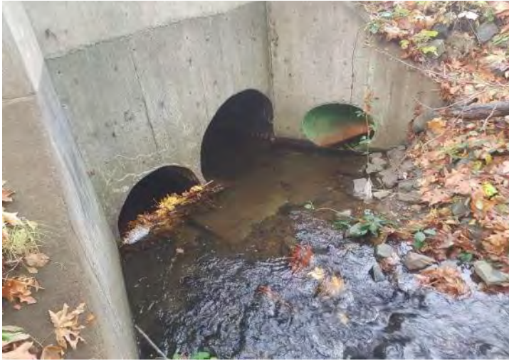
Photo 1, Concrete headwall at inlet.
