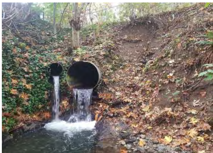
Photo 1, Mild erosion on right bank upstream of culvert.
