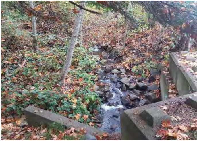
Photo 1, Upstream of culvert with riprap and concrete block wall visible.
