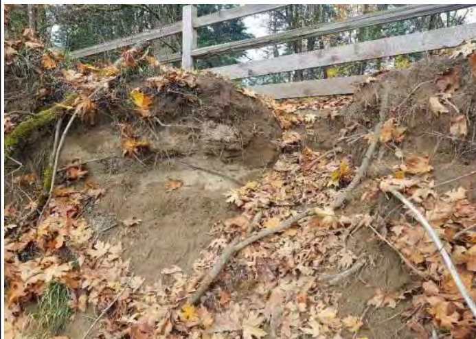
Photo 3, Left bank erosion.
